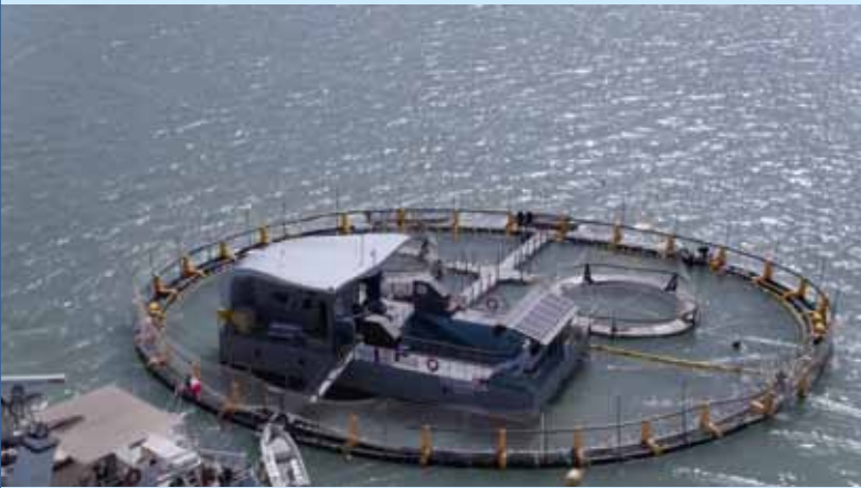
Floating sea pen built for the attempted Vaquita rescue (credit: Terra Mater Factual Studios/Richard Ladkani)
